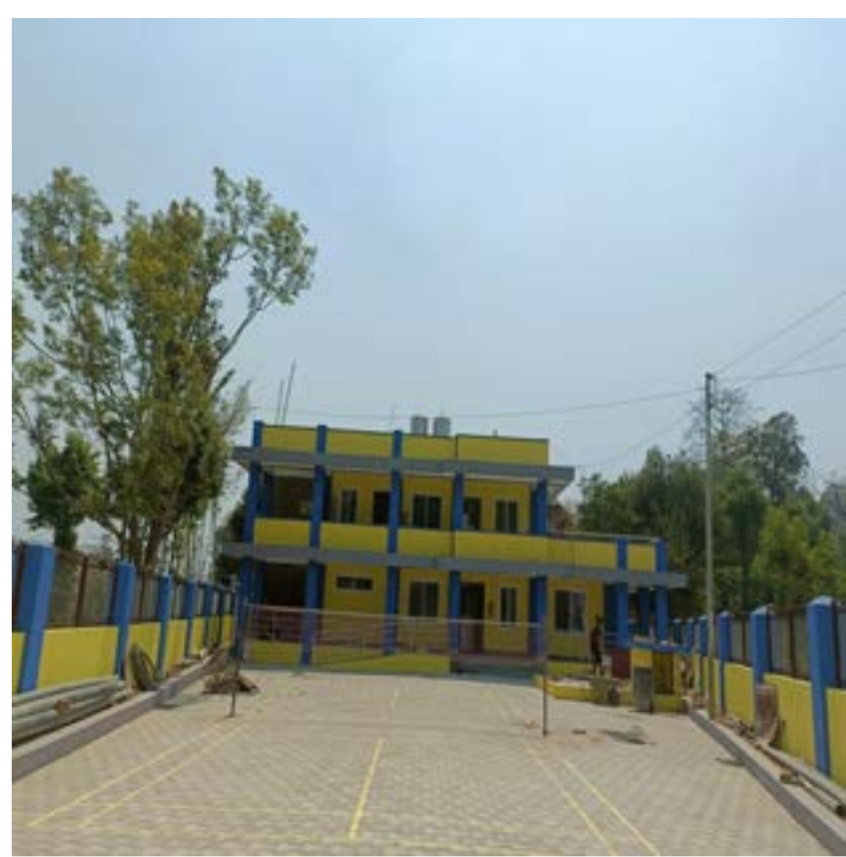
Final Inspection of Health Post Building
